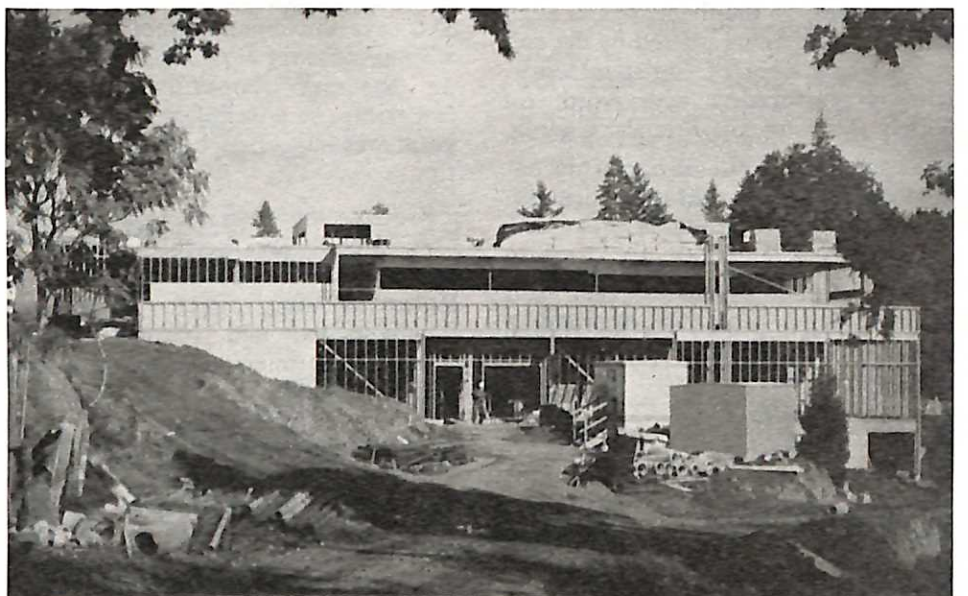
The Coleman Wheeler Sports Center is taking its final exterior shape with four levels visible from the Hess Creek canyon side. The 50,000-square-foot building featuring Northwest lumber products will contain the Miller Gymnasium with three basketball courts, multipurpose physical education rooms, classrooms, and offices for the physical education faculty. The $2.2 million construction project is to be completed spring term.
