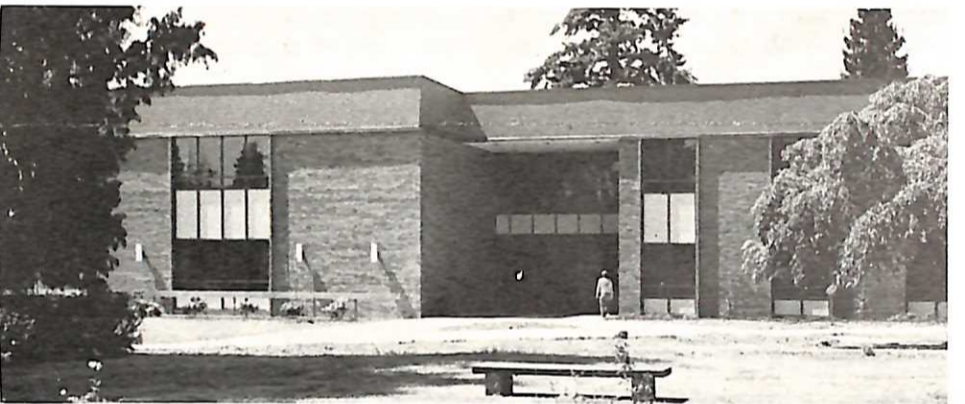
The new Coleman H. Wheeler Sports Center (top), Charlotte Macy and Mary Sutton residence Halls (center), and the Herbert C. Hoover Academic Building (bottom) will be formally opened in a Day of Dedication Oct. 17. The buildings, erected over the last 12 months at a cost of more than $4.3 million, add more than 103,000 square feet of space to campus facilities. Dedication ceremonies will be held at each building, featuring state and national leaders. Public tours of the new buildings are planned.
