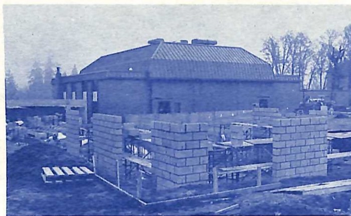
Chapel/Auditorium rises above ground.
