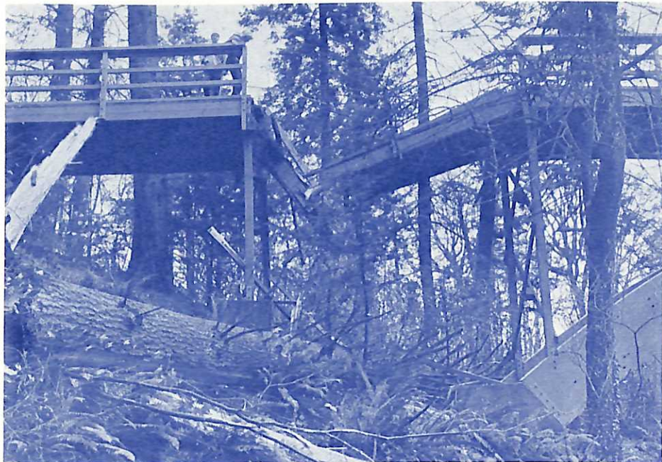
Hess Creek bridge severed in windstorm.
