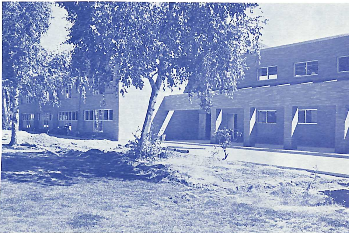
Construction is coming to a close on the M. J. Murdock Learning Resource Center.
