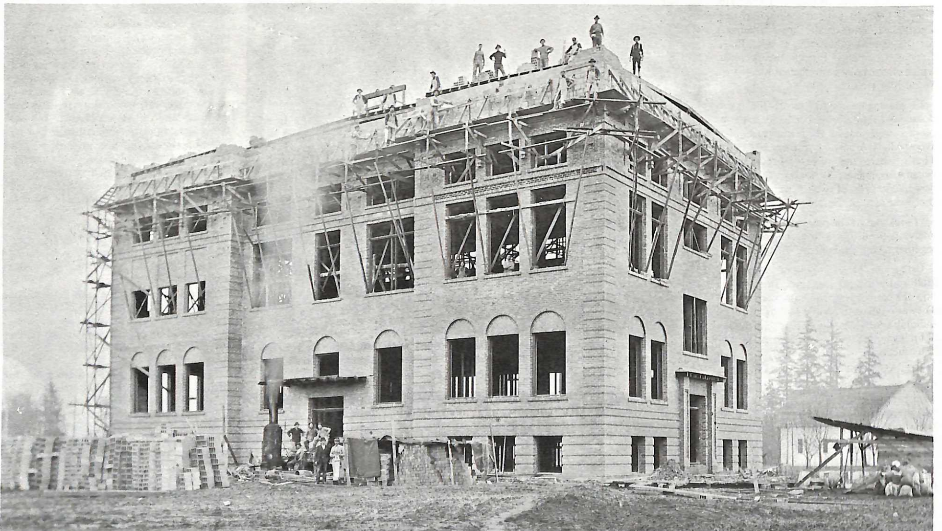
Workers pause to have their photo taken during construction of Wood-Mar Hall in 1910.
