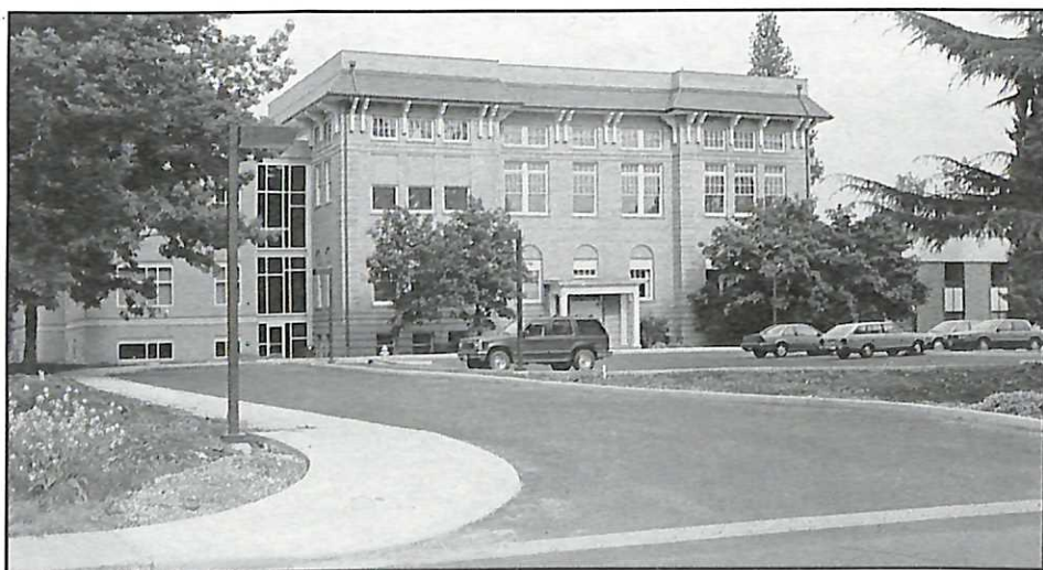
The new main entrance and parking lot is backed by Wood-Mar Hall, which had its Spanish-style cornice restored this spring.
