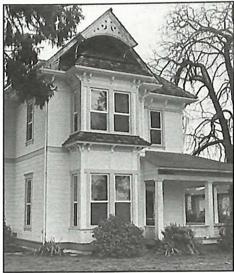
The historic Woodward House in Newberg is the new home for George Fox University's Health and Counseling Services Center.
