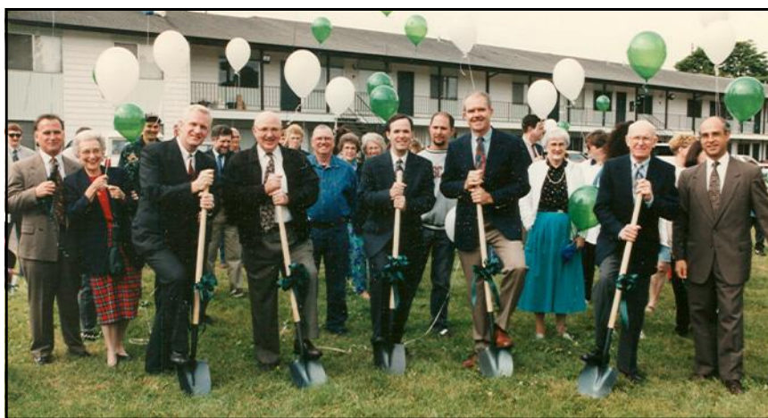
The groundbreaking ceremony for Bristol Hall was attended by many supporters and board members. The men behind the shovels are (L to R) Dennis Lynn, Gene Hinds, Paul Hinds, Randy Young and Lyle Harms.
