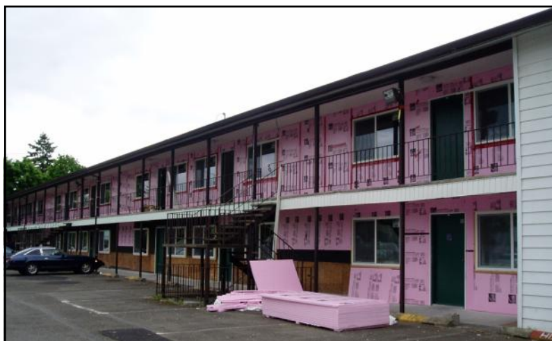
In 2006, the siding was replaced and new windows were installed in Hartzog Hall (the upperclassmen residence hall for women on campus).
