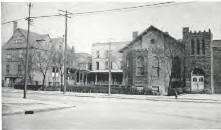
Cedar Avenue Church after remodeling, Soul Winner, and Cleveland Bible College Buildings.
