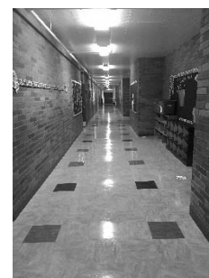
Figure 30: Clean and Well Kept School Building
