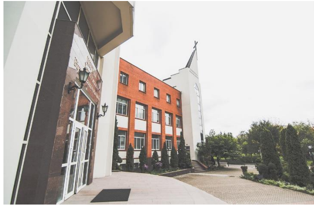
Fig. 18. The Church of Christians of the Evangelical Faith “Philadelphia,” Kiev city, built in 2000
