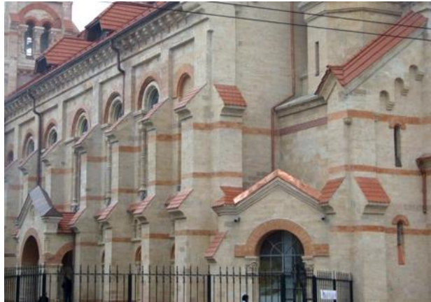
Fig. 9. Neo-Gothic church walls divided into layers by the brickwork. St. Paul Lutheran Church in Odessa
